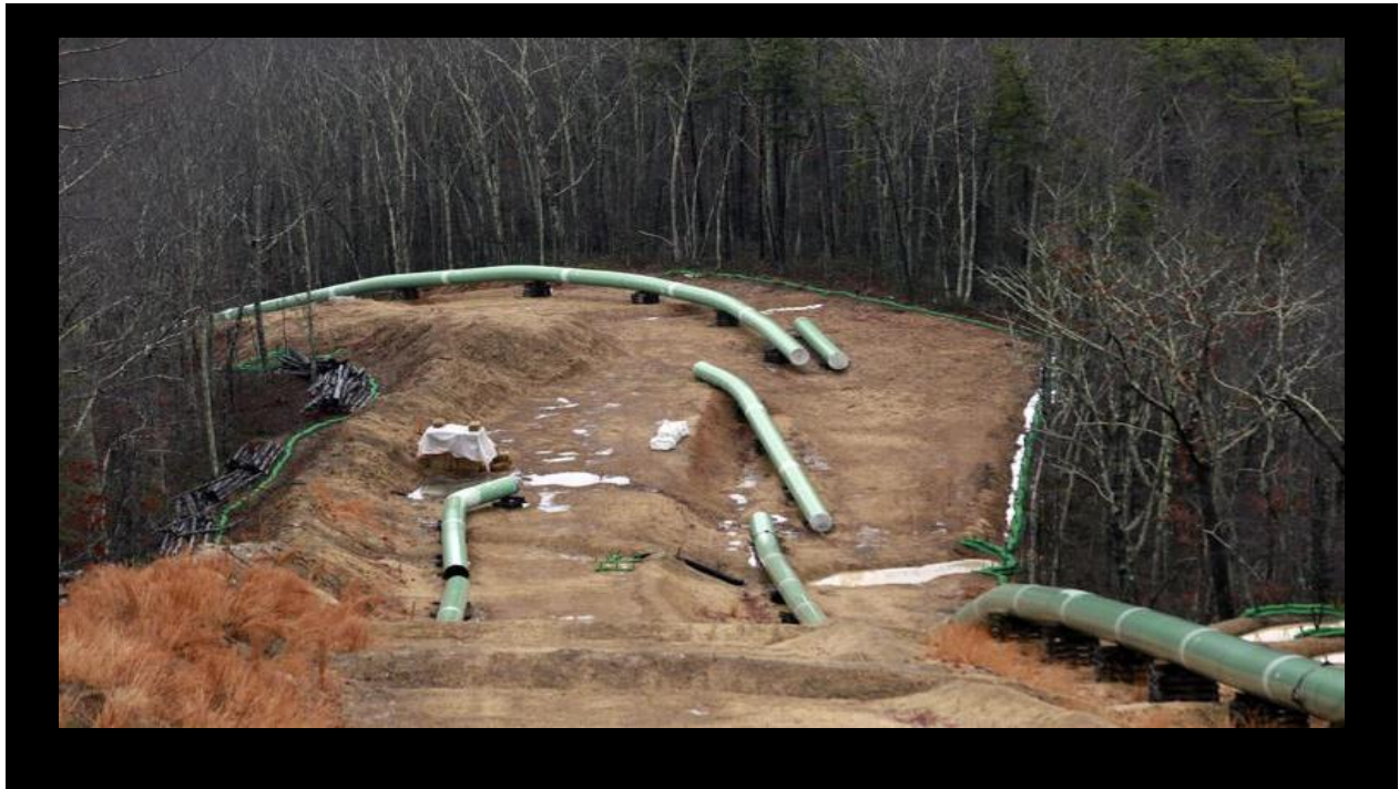
The Mountain Valley Pipeline project's work is seen on Brush Mountain in Montgomery County outside of Blacksburg recently.
