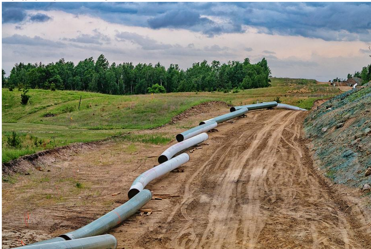
Construction on the Enbridge Line 3 oil pipeline in Northern Minnesota.
