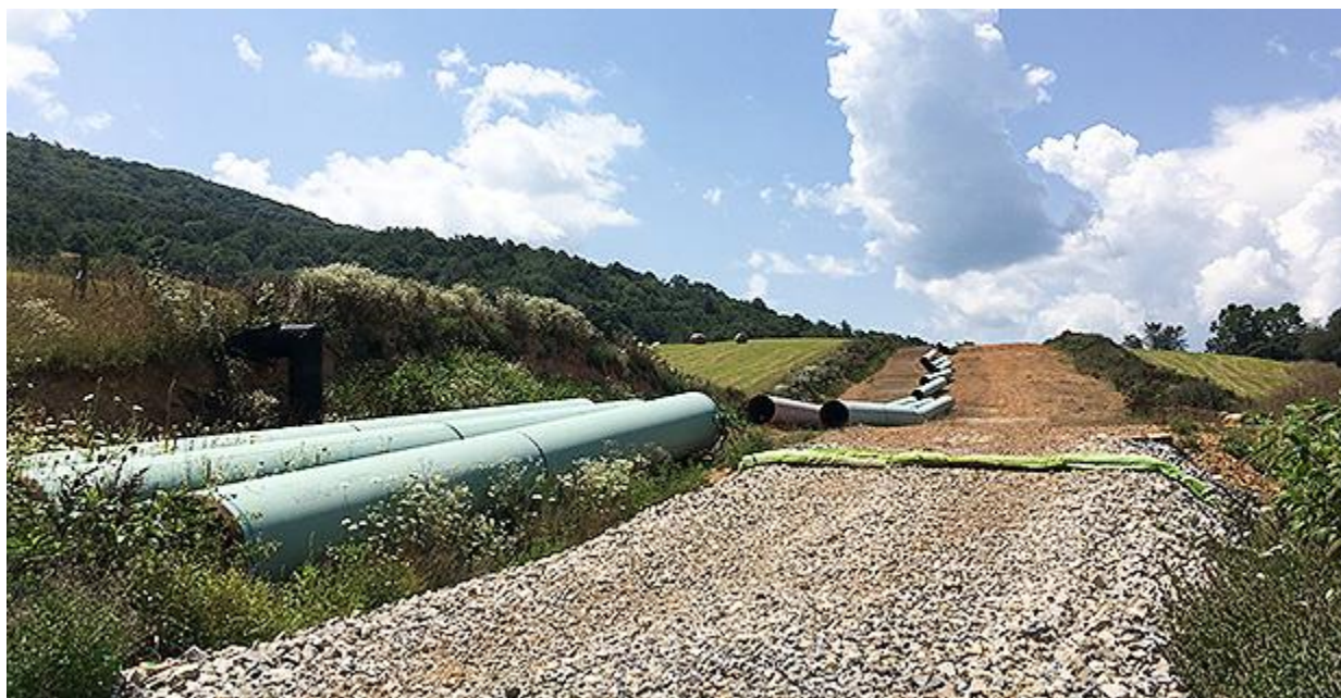
Pieces of the Mountain Valley pipeline awaiting installation in Newport, Va. Pamela King/E&E News
