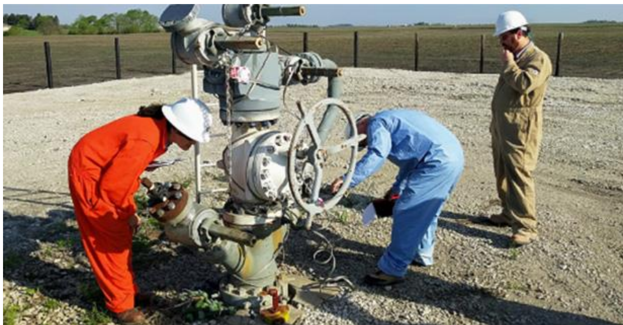
Pipeline and Hazardous Materials Safety Administration employees inspecting a natural gas storage site. Government Accountability Office
