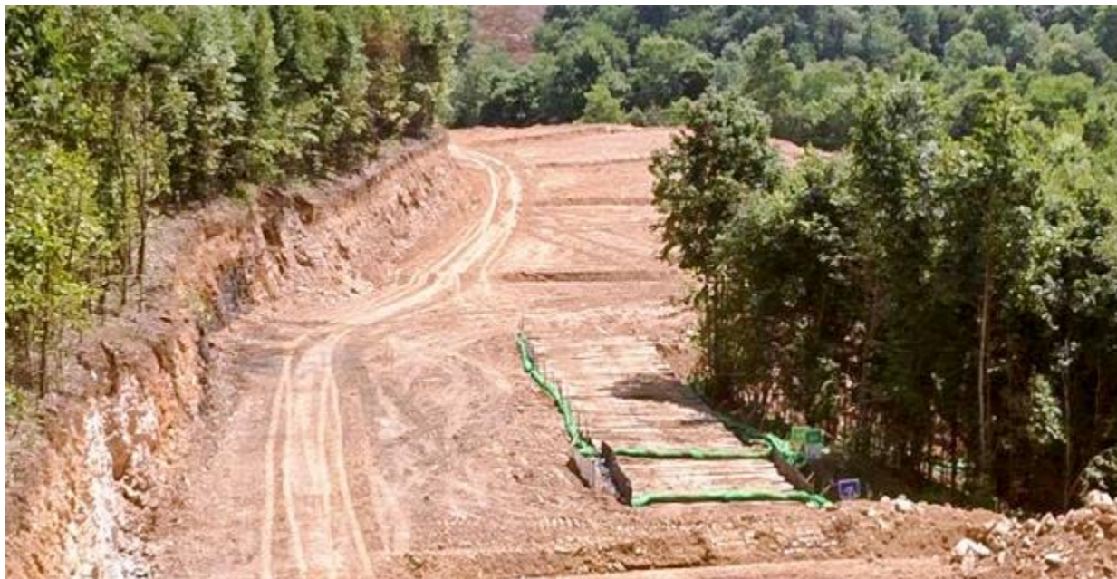
Construction on the Mountain Valley pipeline project in West Virginia is shown. Mountain Valley Pipeline LLC
