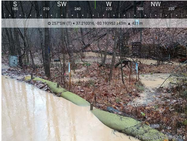
The unnamed tributary (background) running adjacent to Yellow Finch Lane (foreground) feeds into the Roanoke River.
