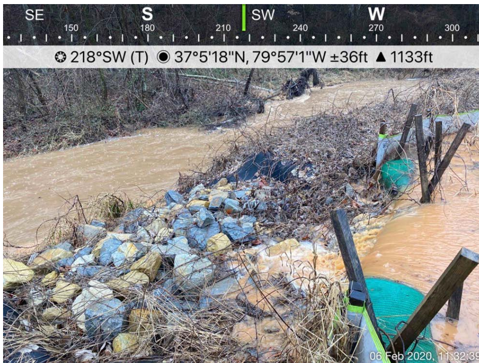
Sediment-laden runoff flowing from the MVP right-of-way over filter socks into Teels Creek, which the 2017 Biological Opinion categorized as “suitable habitat” for Roanoke logperch.
