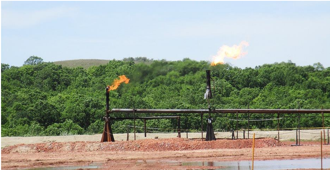
Methane flaring from an oil and gas operation. Interior Department
