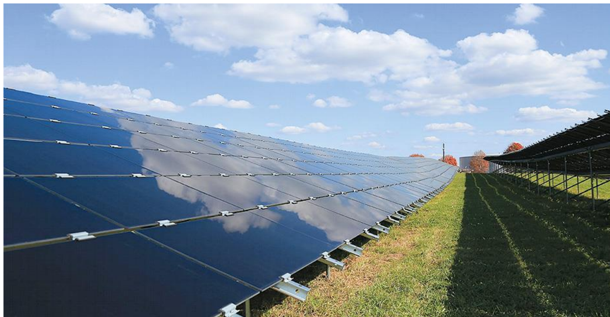
A solar array in Virginia operated by Dominion Energy. Dominion Energy
