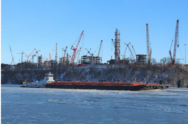
Construction of the Shell Cracker Plant in Beaver County, PA, in January 2019. The plant will be capable of producing 1.6 million tons of raw plastic annually, and is a key development of the new Appalachia petrochemical hub.
