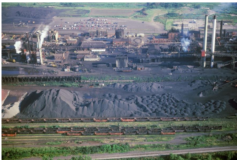
Eighteen coal-fired power plants in Illinois have coal ash dumps that are leaking dangerous levels of toxic metals including arsenic and lead into groundwater – the most of any state in the U.S.
