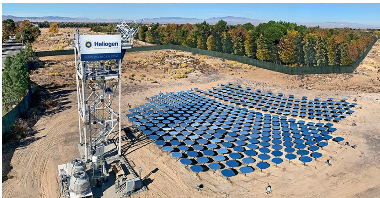
Heliogen's commercial facility in Lancaster, Calif., concentrates solar energy to generate heat in excess of 1,000 degrees Celsius. Heliogen/Business Wire
