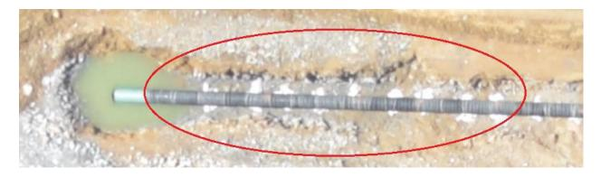
CSI identified 25 locations with large rocks loose in the trench, directly underneath the pipe. (Photo courtesy Allegheny Blue Ridge Alliance)
