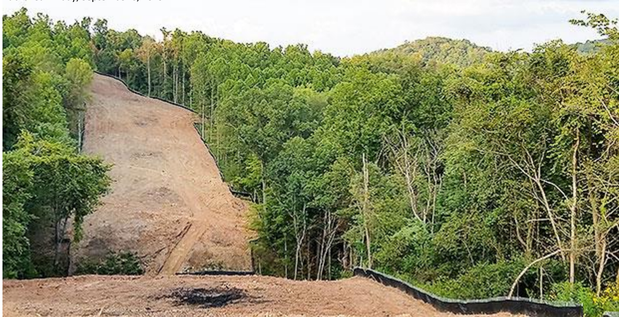
A section of the Atlantic Coast pipeline under construction. Jenny Mandel/File/E&E News
