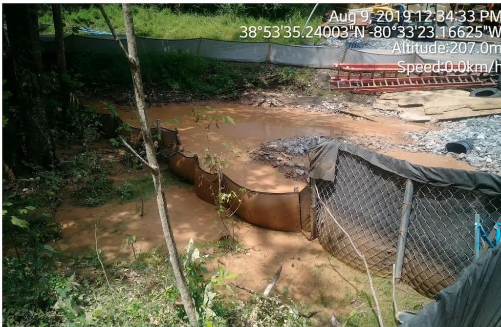
Heavy runoff laden with sediment overwhelms Mountain Valley Pipeline’s sediment and erosion control barriers, making its way into Oil Creek in Braxton County, WV.
