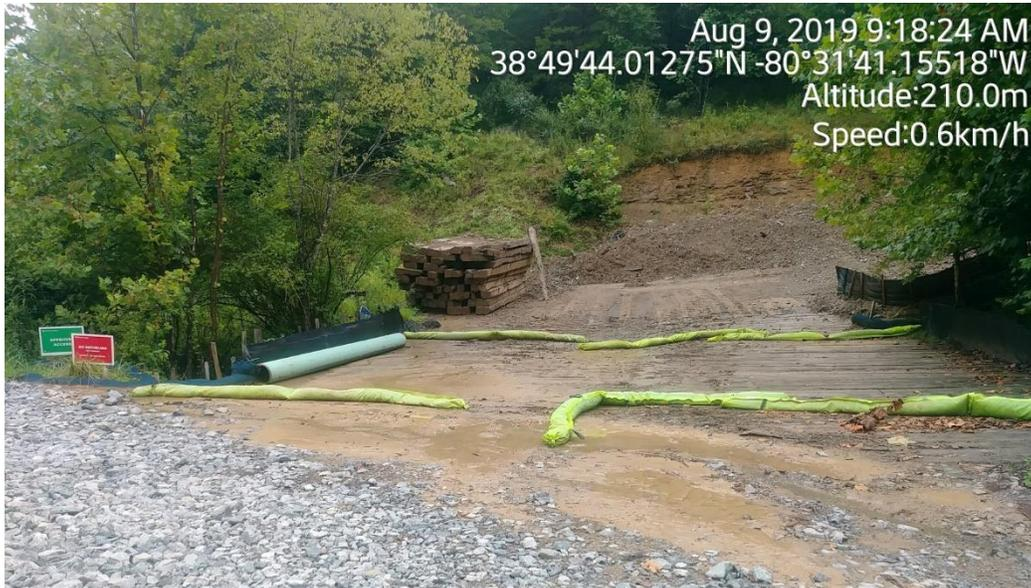
MVP fails to control sediment and sediment-laden water from leaving their access road impacting Barbecue Run which flows into Knawl Creek, a tributary of Burnsville Lake.
