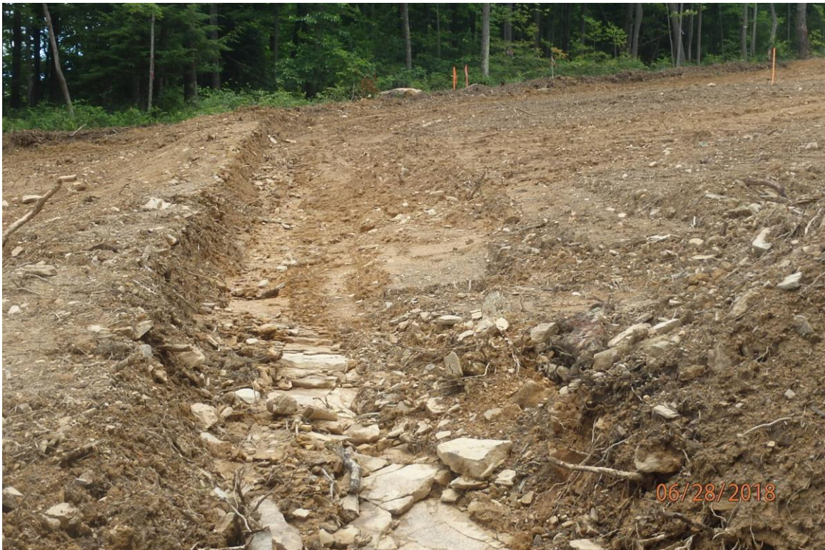
Temporary slope breakers that are installed at a steep angle in the Buckhannon River watershed showing excessive erosion. Deficiencies in site evaluation item numbers 6, 7, 14, 19 & 21 pictured.
