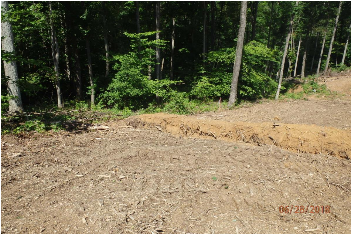
Project area at 1906+00 showing disturbed soil and a lack of treatment at the terminus of the temporary slope breakers and a lack of perimeter silt fence (BSRF) as indicated in the approved SWPPP. Marginal deficiencies in site evaluation item numbers 1, 13, 15, 19 & 21 pictured.
