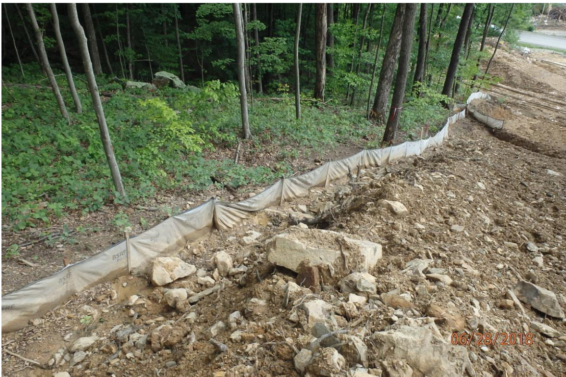
Temporary slope breakers that do not extend past the installed perimeter silt fence from 1789+00 to 1794+00. Marginal deficiencies in site evaluation item numbers 7, 14 & 21 pictured.
