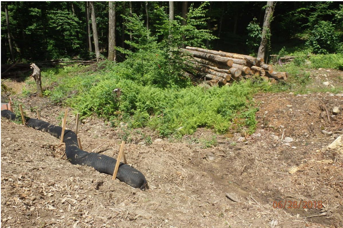
Ephemeral stream adjacent to 1878+00 showing the need for modification of the approved SWPPP for additional BMPs. Marginal deficiencies in site evaluation item numbers 1, 13, 15, 19 & 21 pictured.
