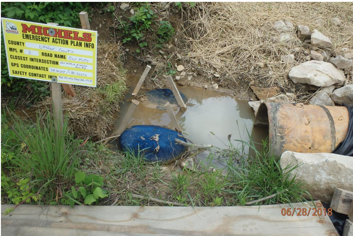
Installed compost filter sock in the roadside ditch along Our Mills Road (1974+61) that is not being properly operated. Deficiencies in site evaluation item numbers 2, 6, 19 & 20 pictured.
