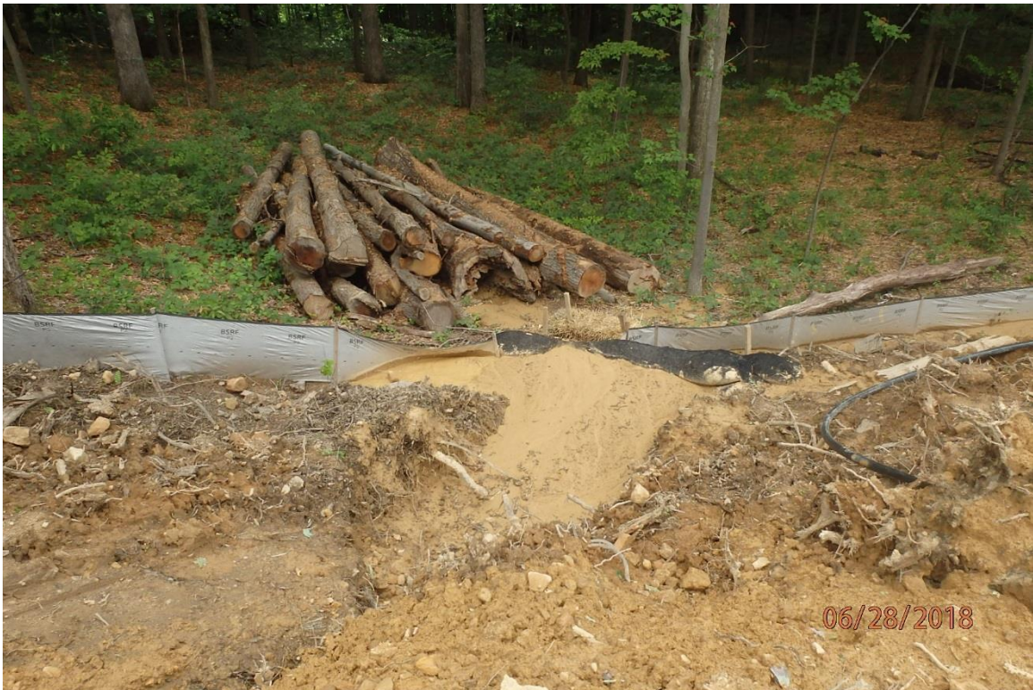
Temporary slope breaker terminus treatment that has been overwhelmed due to excessive erosion at the slope breaker and the associated offsite sediment deposits in the UNT Buckhannon River watershed. Deficiencies in site evaluation item numbers 6, 7, 14, 19 & 21 pictured.
