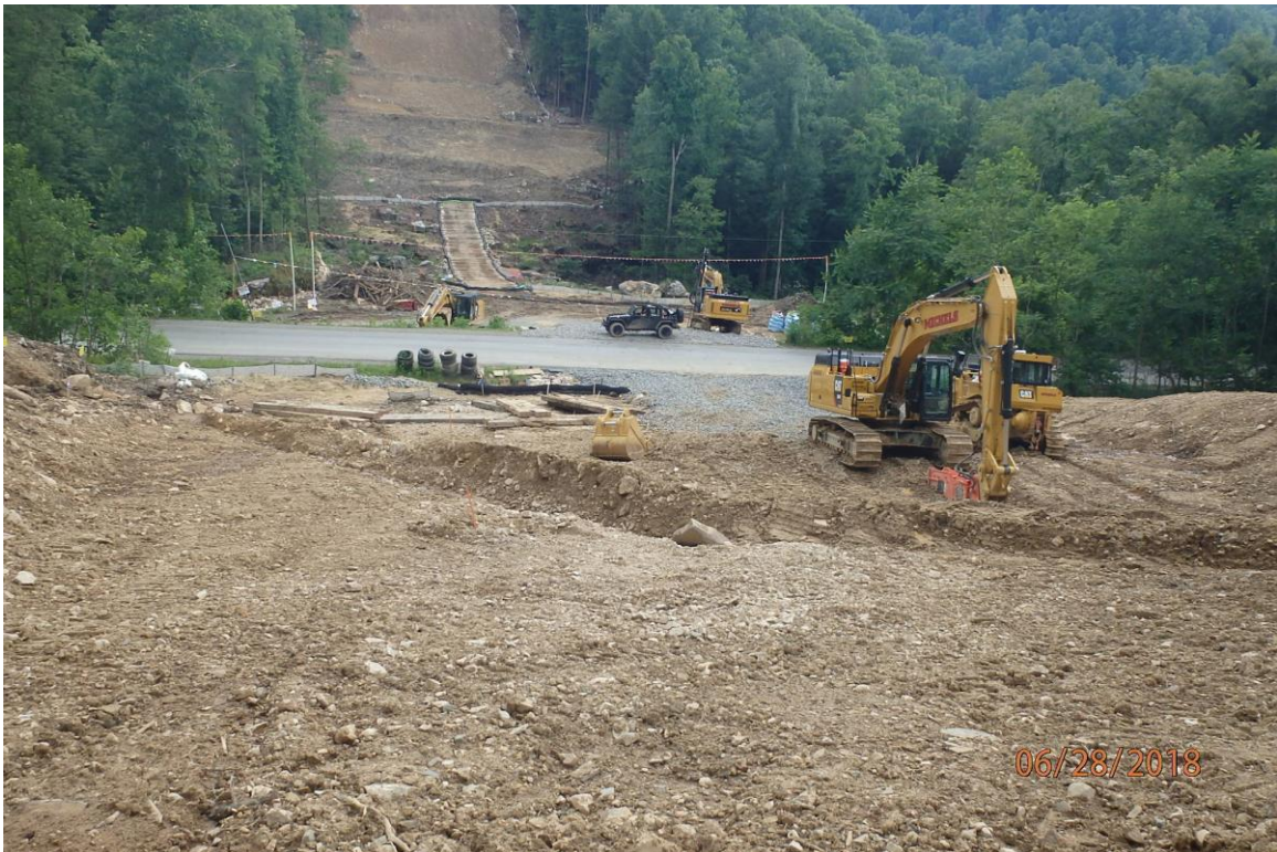
Temporary slope breakers that are installed at a steep angle in the Grassy Run watershed. Deficiencies in site evaluation item numbers 6, 7, 14, 19 & 21 pictured.
