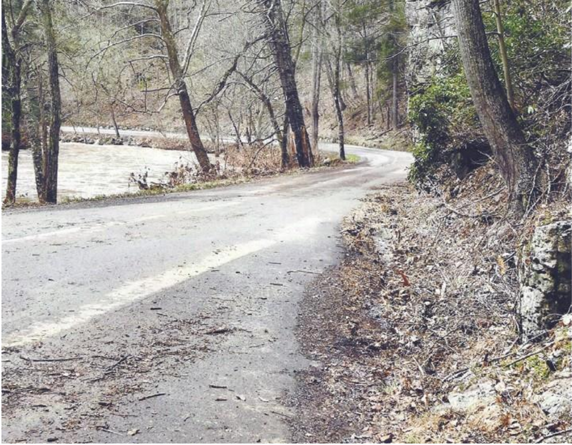
Left: Approaching this sharp turn in the Bullpasture River Gorge, the rock cliff abuts the road and leans toward the road. There is no shoulder across from the cliff, and the bank falls sharply into the river. All photos were taken on April 16,2018. (Photos courtesy PriscillaMelchior)
