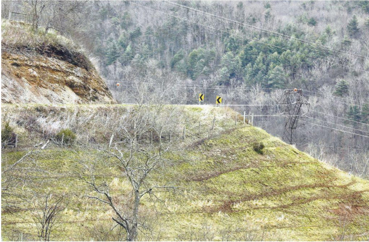
Above: Looking north just past the Shumate house, there is no road shoulder on either side as the road heads up between a steep bank on the left and a larger, extremely steep bank on the right. There is no guard rail and no room for one. At the top of the hill, the road makes a blind, more than 90-degree turn.
