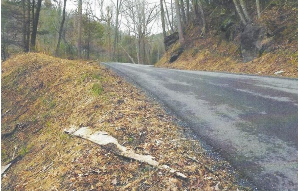
Route 678 rises through the gorge. There are no guard rails, and they would be difficult to install for lack of space in most places. This is one of several blind turns encountered through the gorge.
