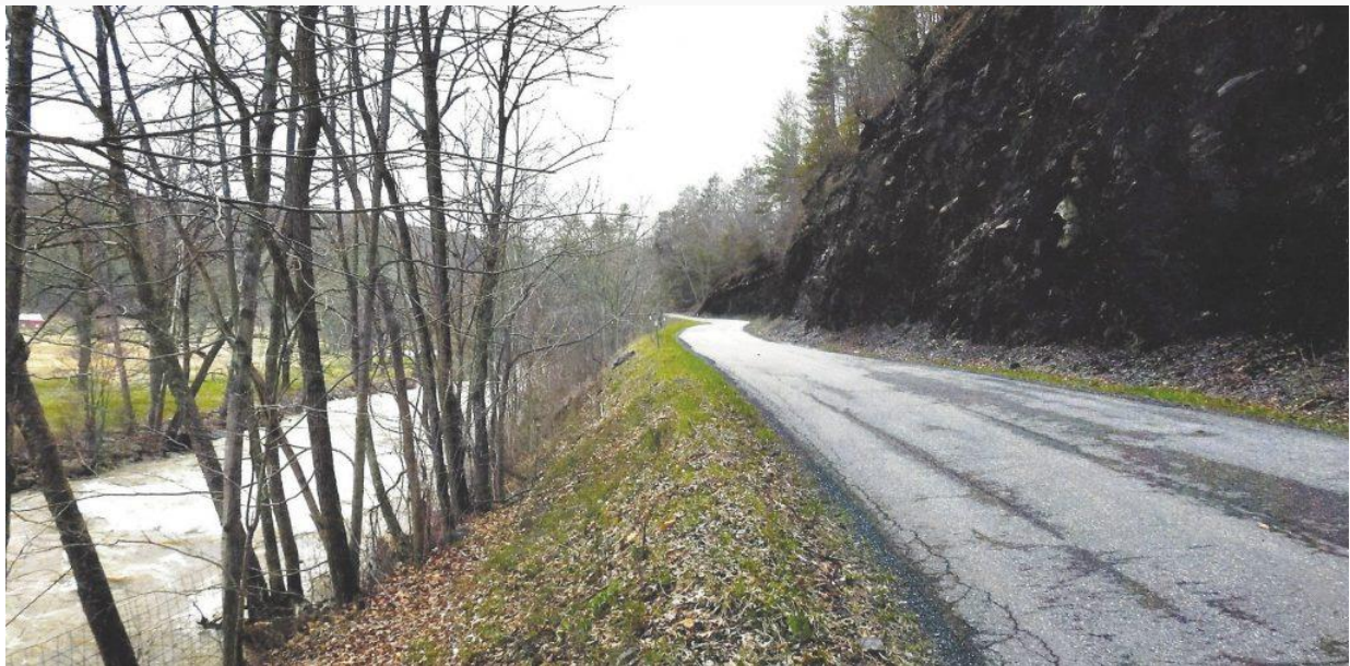
This is the shale bank as seen from the north. There is no shoulder on either side of the road, with the shale cliff on the right, and a steep bank into the river on the left. The cliff frequently sheds rocks onto the road.
