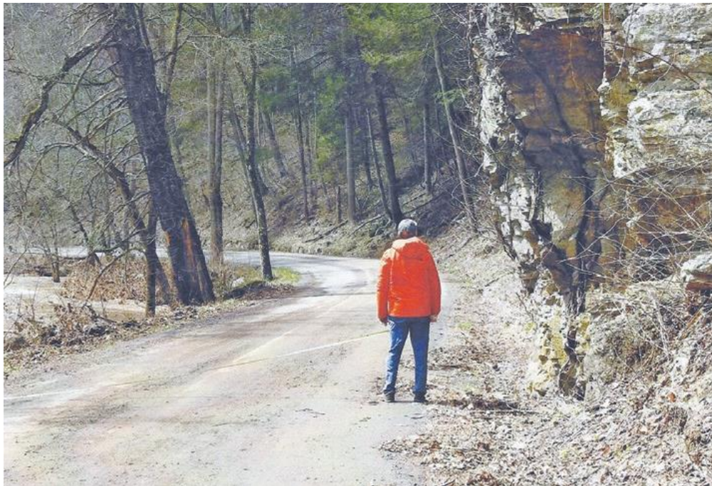
Chris Little measured the width of Route 678 at the rock cliff. His right foot was on the edge of the pavement, which measures less than 17 feet wide.
