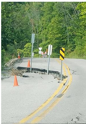
Trucks carrying pipeline and gas production equipment have taken a toll on rural roads like this one in Wetzel County, W.Va., where a caved-in section of blacktop has been marked with road signs to warn drivers of the single-lane conditions. Jenny Mandel/E&E News
