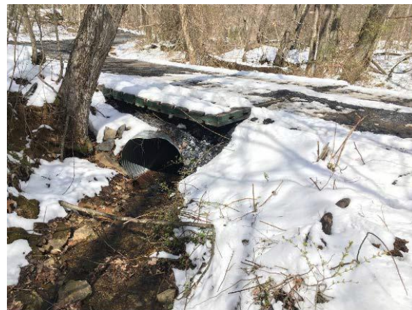
Left: March 23, 2018, Spread 5, MP 157.7, View south of ground disturbance, equipment, and 5-gallon buckets of hydraulic oil by blue tarp not in secondary containment. Right: March 23, 2018, Spread 5, MP 157.7, View north of timber mats and gravel placed over culvert on unidentified tributary.
