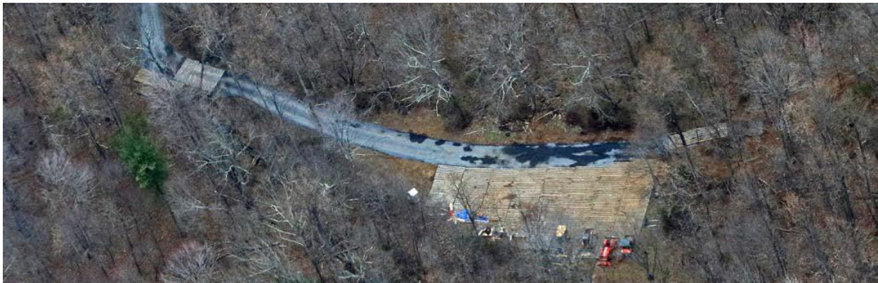
Apparent equipment staging area and new or reconstructed road and bridges observed during Pipeline Air Force surveillance flights. (3/11/18)
