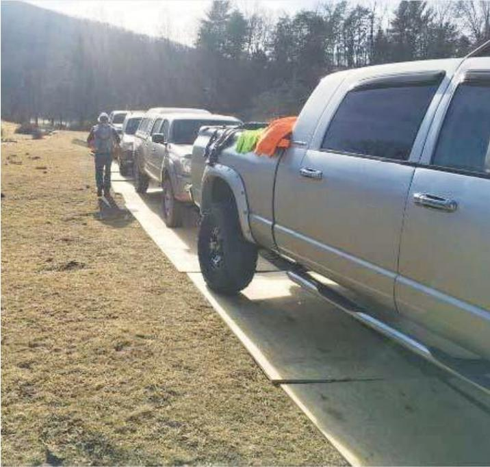
*Plywood was used to prevent rutting by truck tires.*
