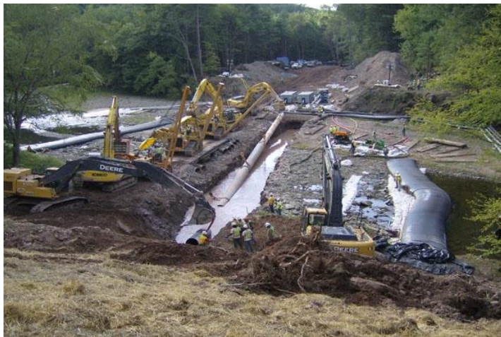
Smaller pipeline than the ACP
