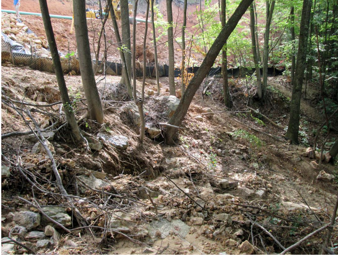
Sedimentation at Columbia Gas Site near Jefferson National Forest (Source: Dominion Pipeline Monitoring Coalition)
