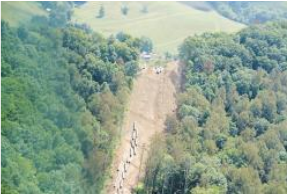
Stonewall Gathering pipeline construction in rugged mountainous terrain, up one side, across the top, and down the other side. This pipeline in West Virginia is 36 inches in diameter. Imagine the pipeline right-of-way on either side of this steep ridge then crosses a narrow V-shaped valley. (Photo courtesy the Dominion Pipeline Monitoring Coalition)
