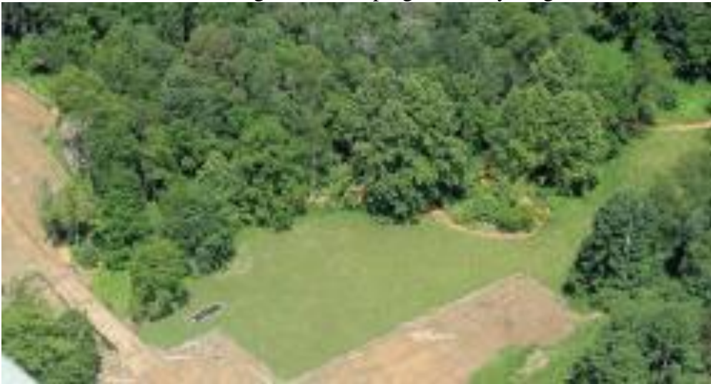
Stonewall Gathering 36-inch diameter pipeline construction in a flat valley with the stream crossing shown in the lower left-hand corner, and heavy stream sedimentation flowing eastward toward the upper right-hand corner. The stream crossing location and extensive construction staging areas are in a flat valley. Observe mud everywhere. What do you think will happen in a narrow, V-shaped valley with steep gradients both east and west? (Photo courtesy the Dominion Pipeline Monitoring Coalition)
