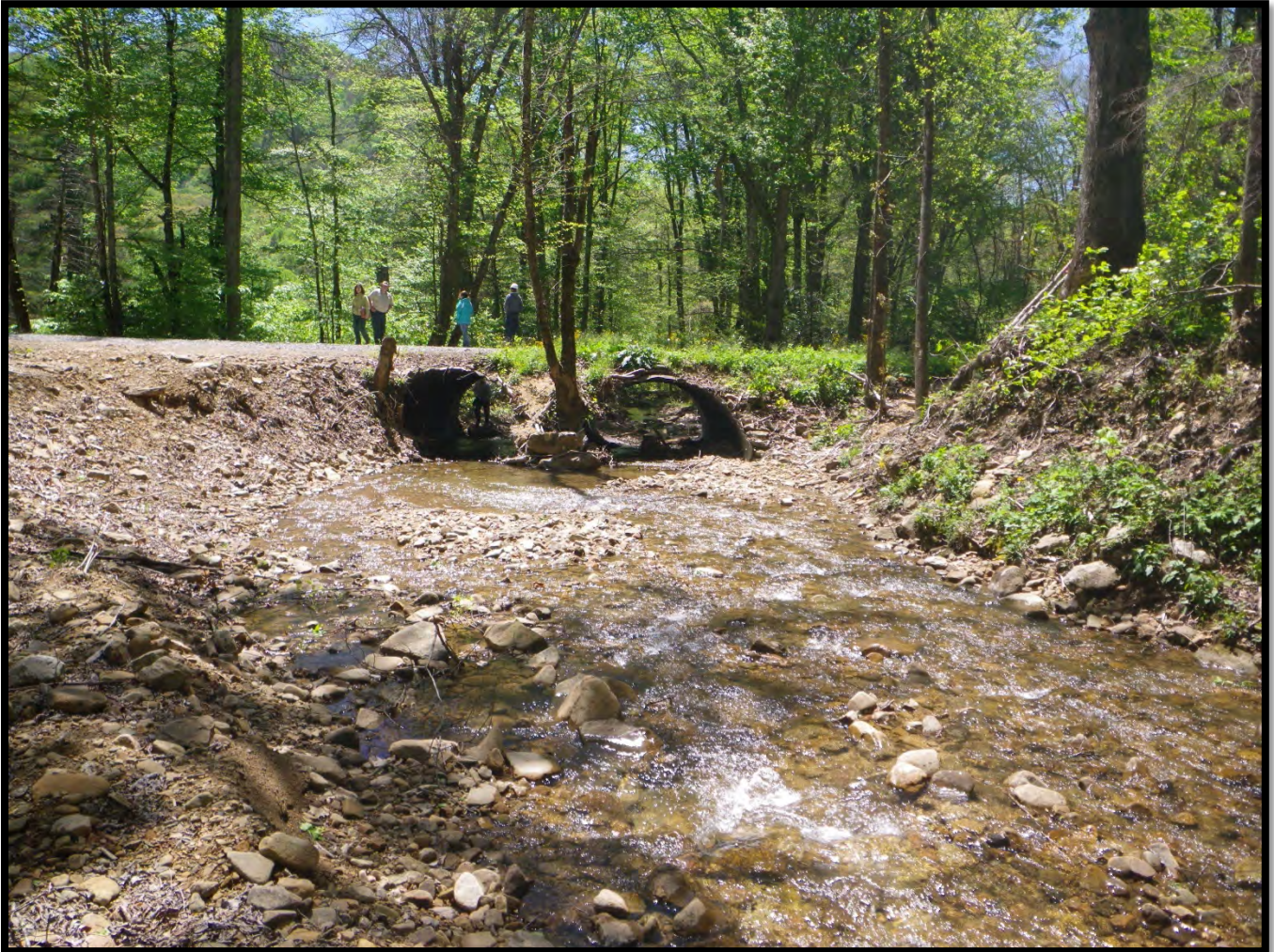
Figure 8. Culverts at Milepost 16.6, Photo Taken 5/3/2017
