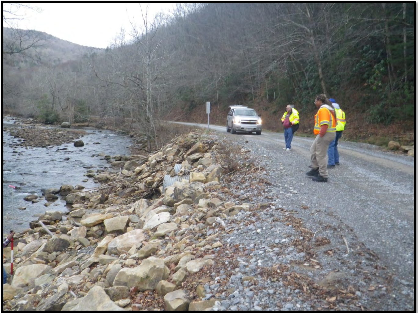
Figure 12. Culverts at Milepost 5.9, Photo Taken 11/30/2017
