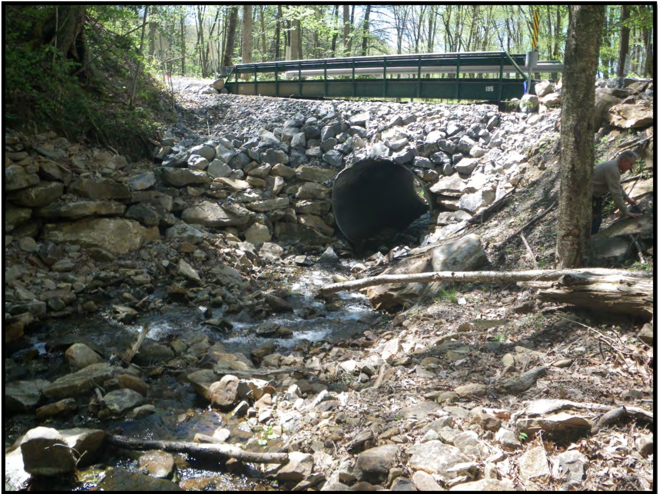
Figure 9. Culvert on FS 133 at Milepost 1.19, Photo Taken 5/3/2017
