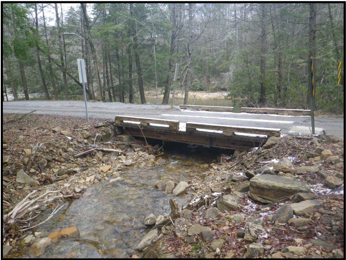
Figure 11. Timber Bridge at Milepost 10.8, Photo Taken 4/10/2018
