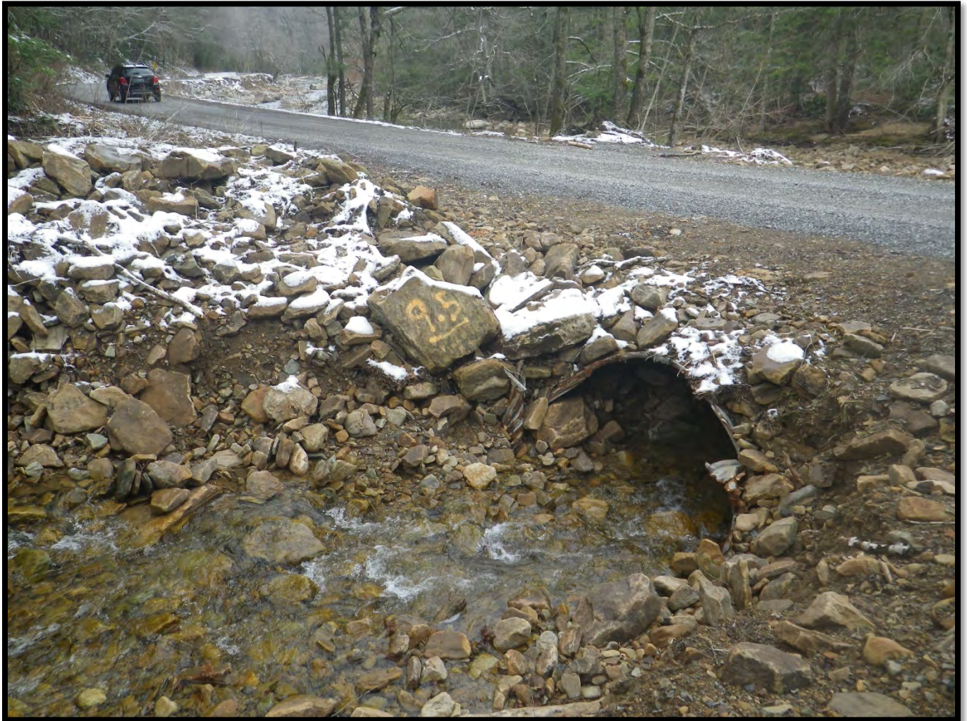
Figure 10. Culvert at Milepost 9.5, Photo Taken 4/10/2018
