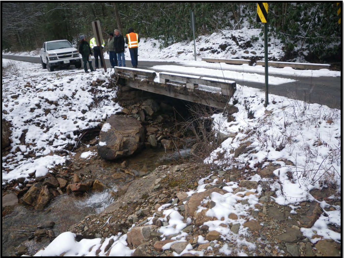
Figure 13. Timber Bridge at Milepost 6.7, Photo Taken 4/11/2018
