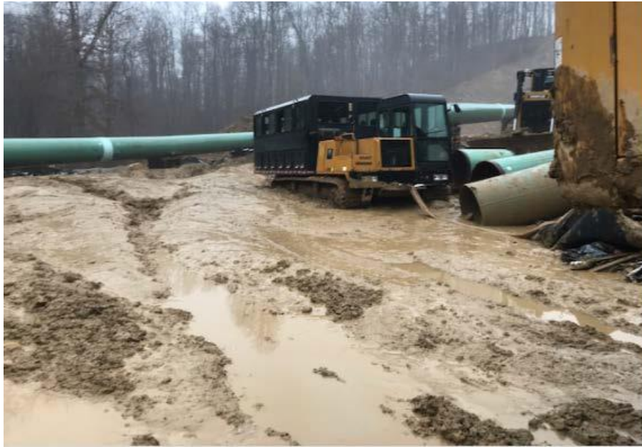
Spread 2-1, MP 40.1, View west of Marooka stuck in mud and liquified soil.
