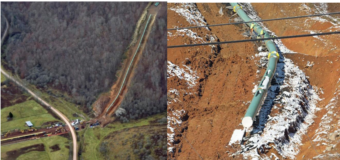
Above left: Pipeline Air Force photo of ACP construction in Dry Branch and Middle Mountain area in Pocahontas County. Above right: Citizen volunteer observer photo of ACP construction on Middle Mountain in Pocahontas County. In both instances, water bars had not been installed as required for steep slope construction.
