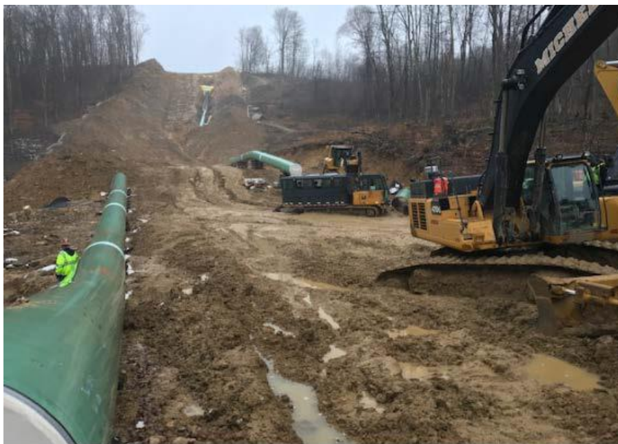
Spread 2-1, MP 40.1, View north of mud and liquified soil in travel lane. Note depth of mud over equipment tracks.
