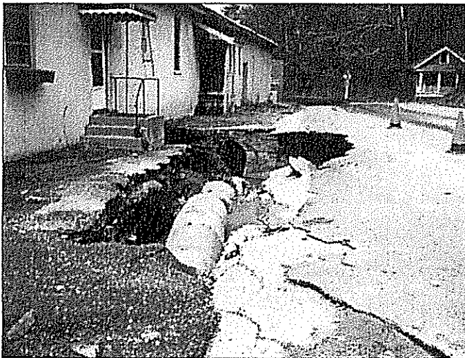
The road in front of The Homestead purchasing office was washed out. (Photo courtesy Bath County Historical Society)
