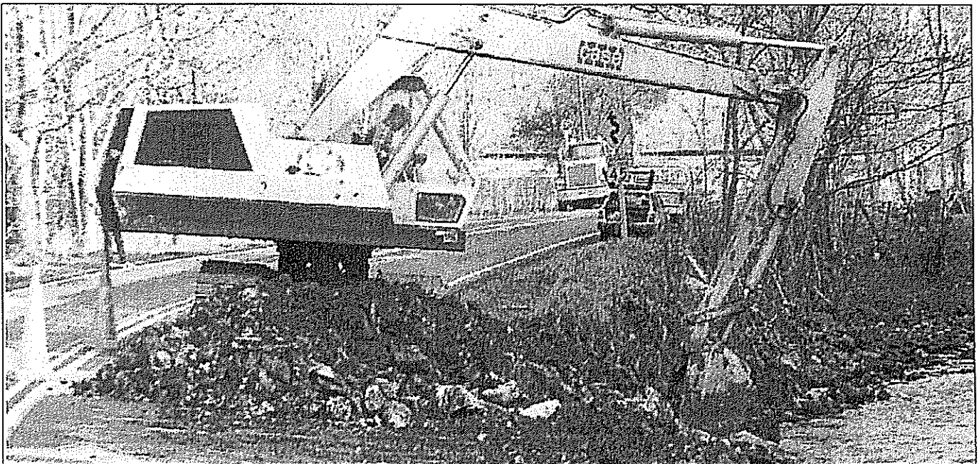
Pictured is the bank of the Jackson River being rebuilt after the flood. Plecker and Sons Excavating of Millboro dumped tons of fill rock in the area along U.S. 220 south of Mustoe that was washed out by the flooding. (Recorder file photo)
