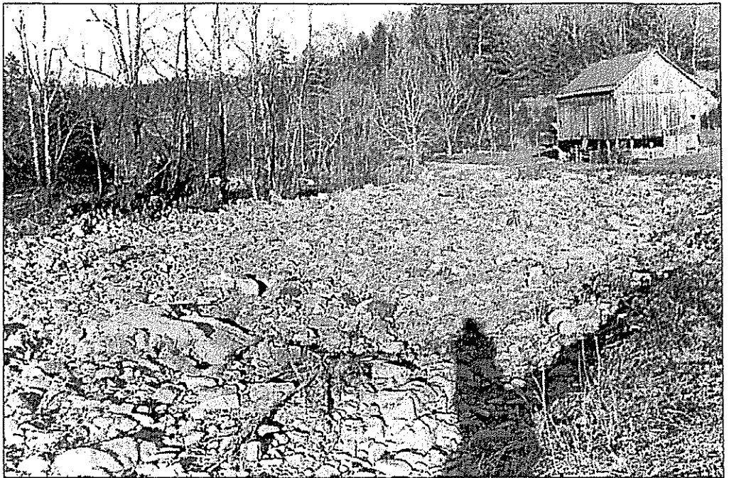
The Cowpasture River deposited tons of river rocks on Route 614 north of Williamsville. The sudden force of the often dry river moved the road from the tree line on its banks into an alfalfa field and took an untold amount of fence and pasture with it. (Recorder file photo)
