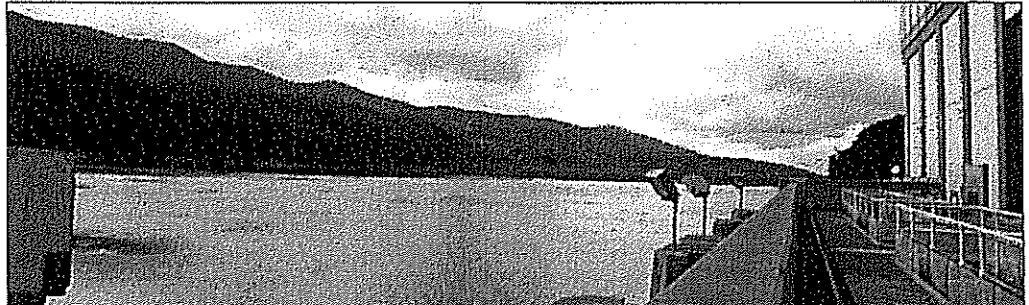
The lower reservoir as seen from the deck of the power station. There is also an upper reservoir, and Veeco built two dams, one for each body of water. (Recorder file photo)
