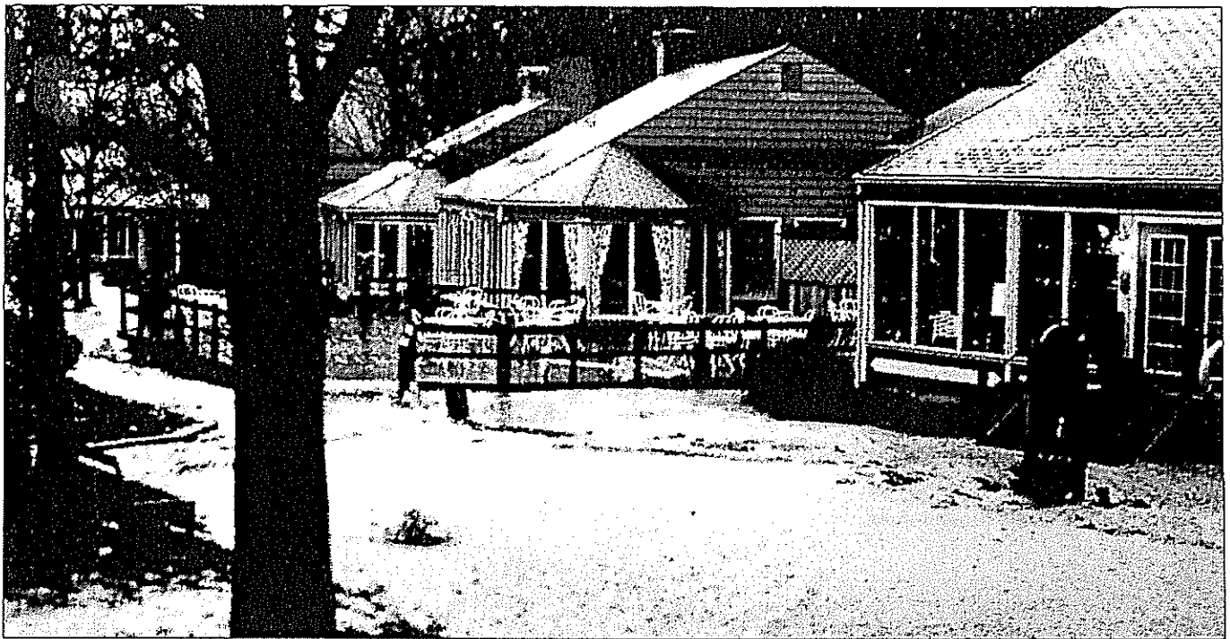
Cottage Row at The Homestead was under water during the flood of 1985. (Photo courtesy Bath County Historical Society)
