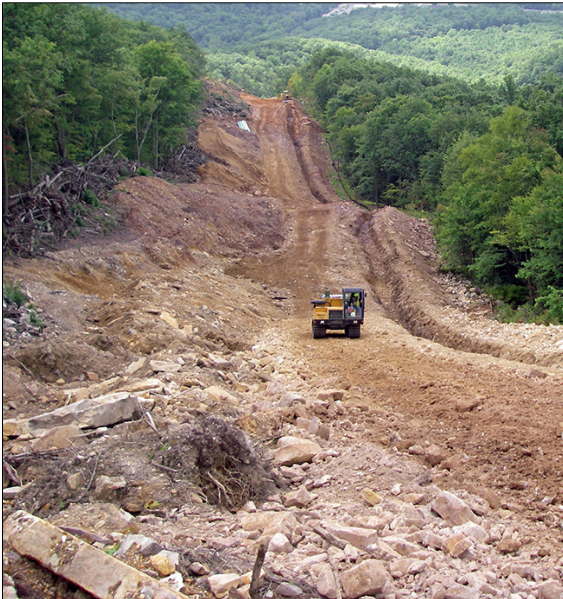
FIGURE 14 – A comparatively small 2014 pipeline replacement project in the Jefferson National Forest on Peters Mountain in Giles County, Virginia. A variance to the 500-foot open trench limit was requested for this project. Although slopes exceeded 40%, the DEQ approved the variance request, allowing a 2,000-foot open trench. No water interceptor diversions were installed during trenching. Following a rain event that occurred shortly before the above photo was taken, a Forest Service employee described having “never seen that much sediment move off site before.” A case study report is posted at www.pipelineupdate.org/case-study-no-1/ . The Dominion Pipeline Monitoring Coalition has conducted a study of open-trench variance requests for pipeline construction projects in Virginia. Fifteen variance requests were submitted between January 2011 and July 2014, and all were approved. The authorized open-trench lengths ranged between 800 feet and 15 miles, with an average length of 2.3 miles.
