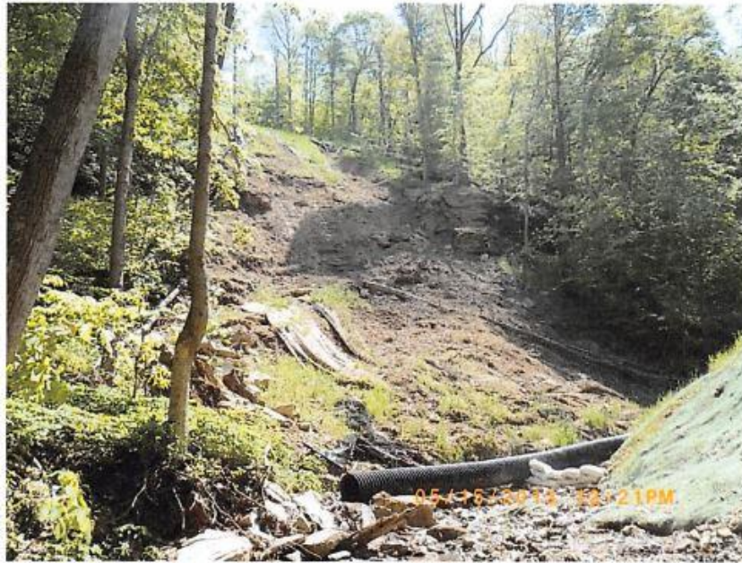
Photo 3: N 39° 52.3772' W 80° 41.1271' Bartletts Run. Flume pipe, sand bags and slip material in stream.
