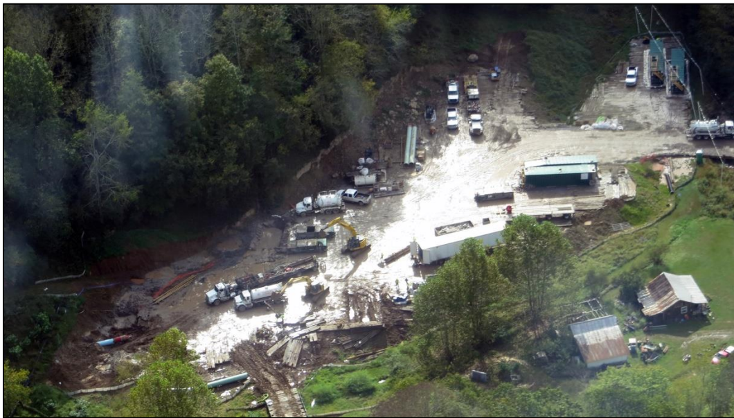
FIGURE VII(c) – Entry-side workspace for a comparatively small HDD operation for the Stonewall Gathering Pipeline in West Virginia. The pullback phase has been completed and the drilling rig has been removed. This operation involved a 1,000 foot boring to install a 36-inch pipeline under Interstate 79.
