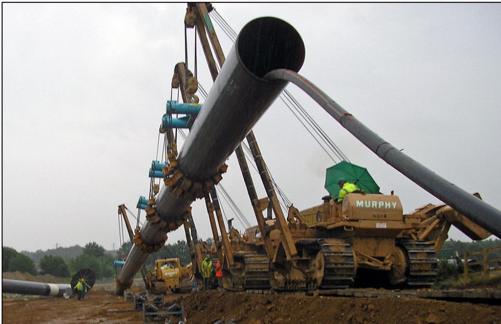
FIGURE VII(e) – Extreme pullback required for the proposed Blue Ridge HDD.
