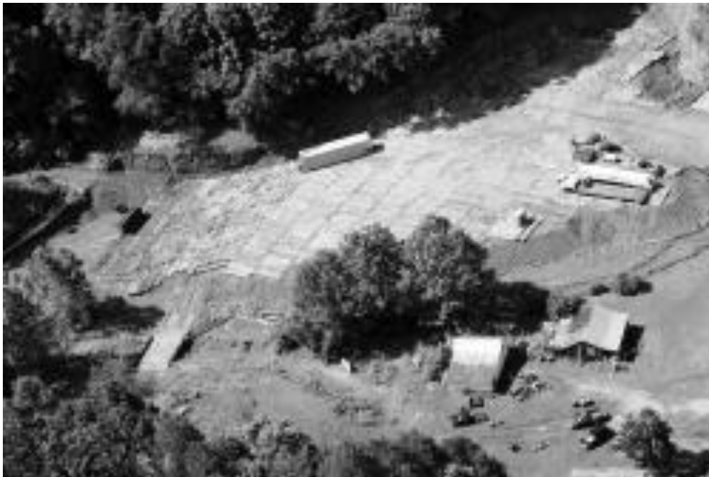
The Pipeline Air Force, part of Dominion Pipeline Monitoring Coalition, took this photo showing the staging area for horizontal drilling under I-95 in West Virginia for the Stonewall Gathering pipeline, which is smaller than the proposed Atlantic Coast Pipeline.
