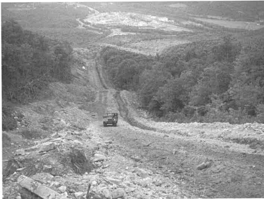
Figure 6. Example of construction road with adjacent pipeline trench. Material excavated for the road is piled on uphill side of road; material excavated for the trench is piled in a berm on downhill side of trench.
