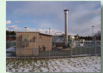
Metering and Regulating Station
